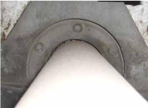
The retractable soot blower port opening will often have a gap, ranging in size from 1/8 inch to 1/4 inch (sometimes larger) allowing leakage. That leakage results in housekeeping issues and localized corrosion.
