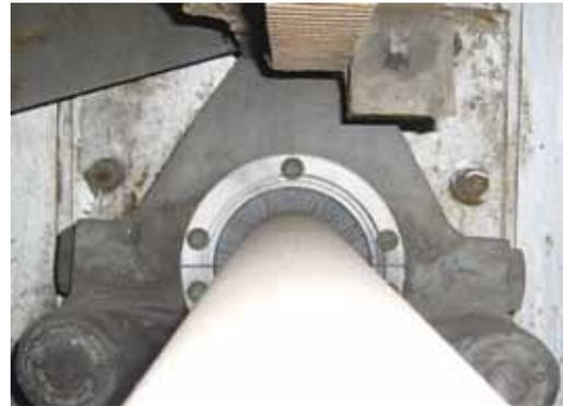
The [Sealeze Adaptive SB Brush Seal](#) is an annular high temperature brush seal that closes the gap while allowing unrestricted motion of the lance tube, minimizing leakage, improving housekeeping and minimizing local flue gas condensation corrosion.
